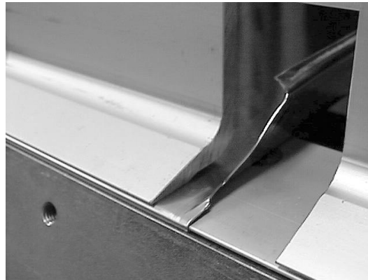
Detail picture step 7. The notch out, should not be more then 25 mm (1")
